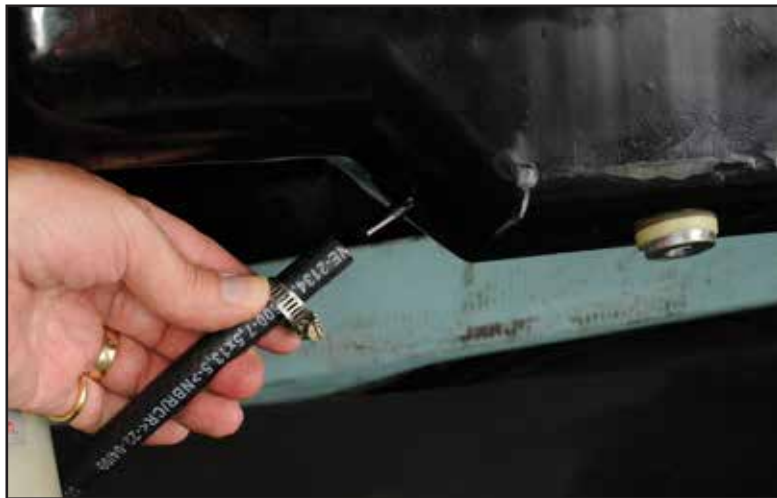
17. Hook new fuel line to gas tank
